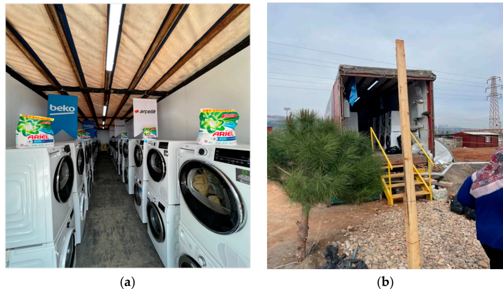
Figure 7. (a,b) Truck with 30 washing machines and 30 dryers for laundry (installed by a private company).
