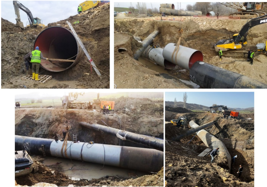
Fig. 20 Replacement of the damaged sections of the water pipe crossing the NG pipe (Courtesy of Gaski)
