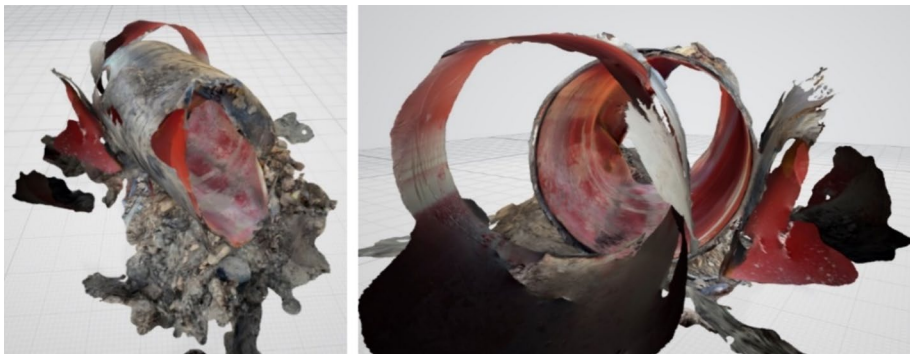
Fig. 19 The 3D Lidar views of the damaged pipe wrinkling (See lidar files #SF6 and #SF7)
